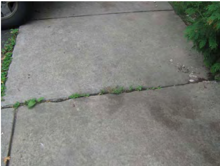
Isolated uneven and cracked section of concrete walkway.
