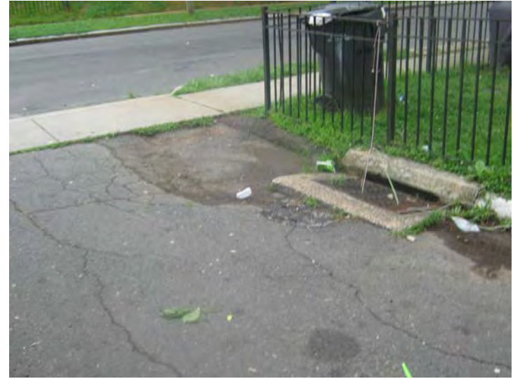
Depressions noted within the asphalt paved surfaces.
