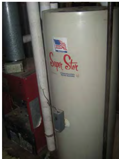
Super Stor indirect fired hot water storage tank – 1 storage tank per unit.
