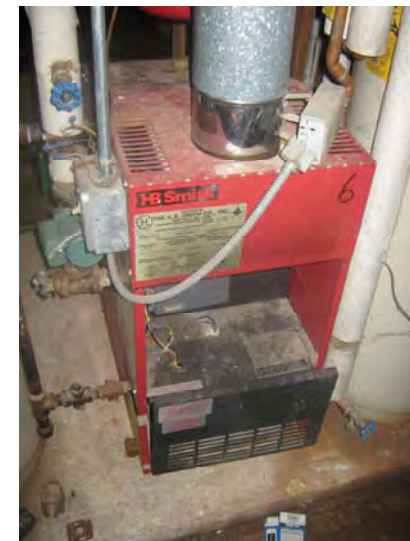
HB Smith boilers for production of hydronic heat – 1 natural gas-fired boiler per unit.
