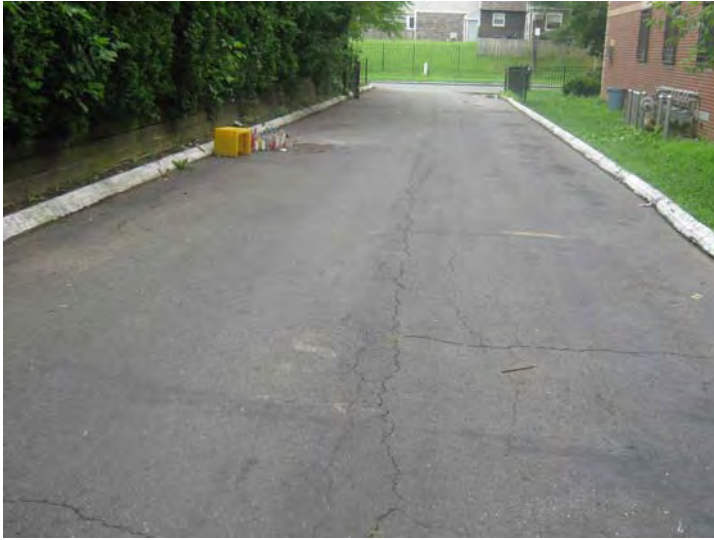
Cracking noted within the asphalt paved surfaces.
