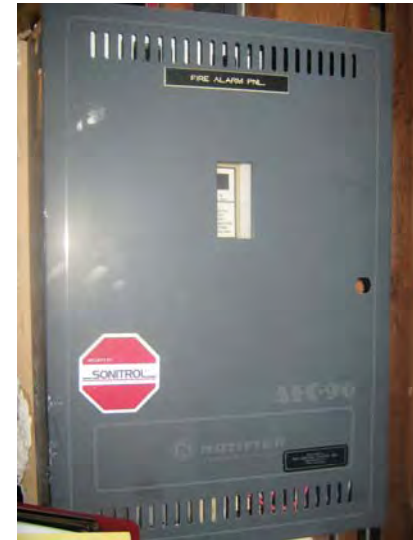
Original fire alarm control panel monitors and supervises hard wired end devices.
