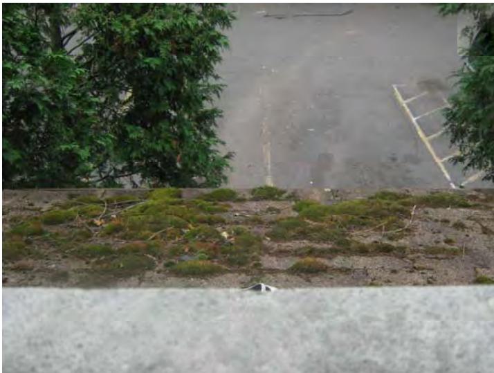
View of widespread moss growth on roof surface at rear entrance/exit canopy.
